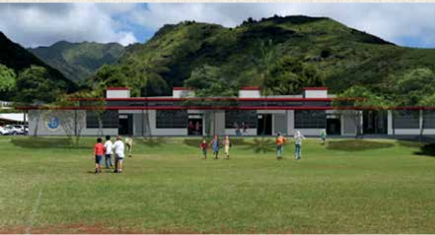
S&M Sakamoto is GC on the high-performance World Languages building at Niu Valley Middle School.
